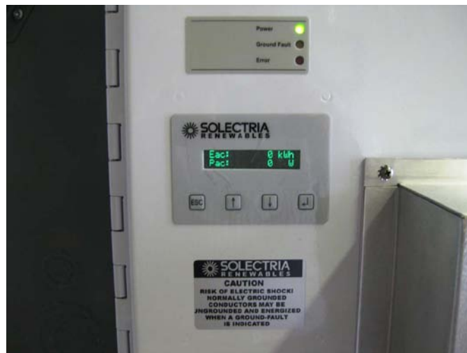
Fig. 7 Front view of inverter showing LED indicators, LCD display and ground fault warning label
