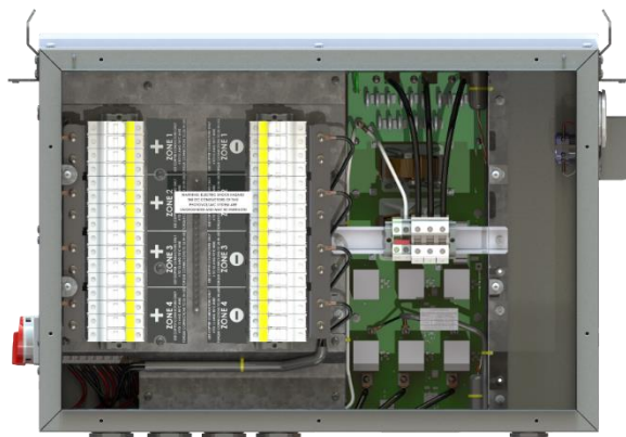
Figure 9-1 Standard Wiring Box
