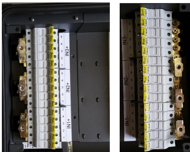
Figure 3-16 Fuse Bypass Kit Installed in the PVI-50-60TL (3 MPPTS)
