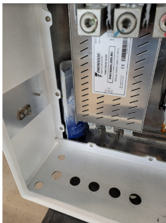
Figure 3-18 Proper Location and Orientation Options for the Desiccant Pack
